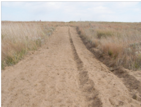
Example of well-constructed disked firebreak.
